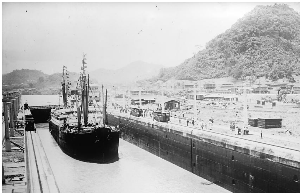
Figure 6.10. Pedro Miguel Locks, Panama Canal, circa 1909-1919. Courtesy The Library of Congress, LC-DIG-npcc-19356.
